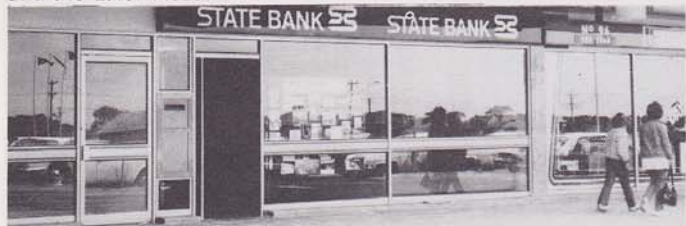
Deer Park: Located one door from Safeway, this branch has four tellers positions and a private interview room.
